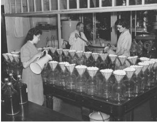
In 1949, labs had to make their own culture medium, a laborious process. In this picture, the man is stirring broth in a vat while the women filter the broth into smaller bottles. After HeLa, it became possible to order ready-made media by mail. © HULTON-DEUTSCH COLLECTION/CORBIS
