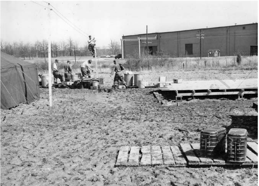
Work detail at Camp USAFOX, aka "Mud." U.S. Army/Courtesy Richard Mitchell.
