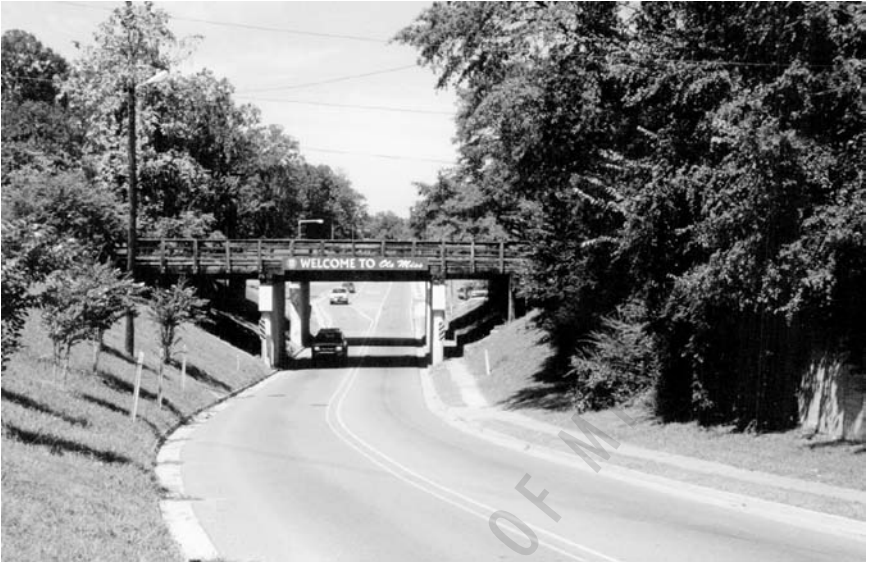
Railroad overpass (since dismantled). At this overpass, a stalled convoy of a unit from the 503rd MP Battalion was attacked by a mob throwing debris from above. Author's collection.
