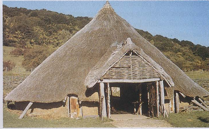
A reconstructed Iron Age farm. Farms like this were established in southeast Britain from about 700 BC onwards. This may have been the main or even only building; large round huts increasingly took the place of smaller ones. "Their houses are large, round, built of planks and wickerwork, the roof being a dome of thatch," wrote the Greek philosopher Strabo. In most of Celtic Europe huts were square.
