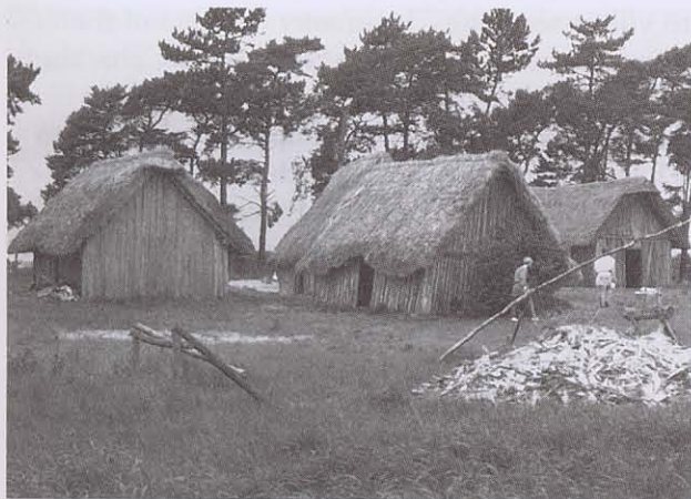
Reconstruction of an Anglo-Saxon village. Each house had probably only one room, with a wooden floor with a pit beneath it. The pit may have been used for storage, but more probably to keep the house off the damp ground. Each village had its lord. The word "lord" means "loaf ward" or "bread keeper", while "lady" means "loaf kneader" or "bread maker", a reminder that the basis of Saxon society was farming. The duty of the village head, or lord, was to protect the farm and its produce.
