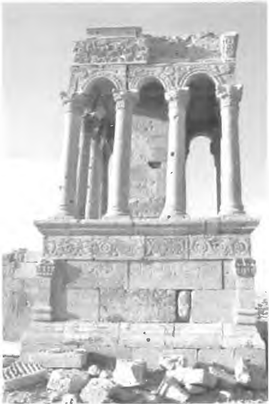
FIGURE 9.4 Detail of temple tomb NC, showing original position of reliefs on the arcade arches and on the frieze above. The surviving fragment of the frieze shows (left) the harvesting of cereals and (right) a hunting scene. (Photo: ULVS.)
